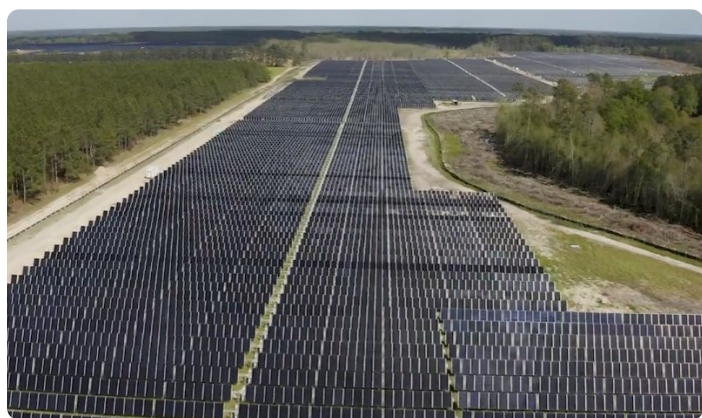
Banc of California helped finance the Snipesville III Solar Project in Georgia, which will provide low-cost, clean energy for generations. The facility can power up to 18,000 homes a year.
